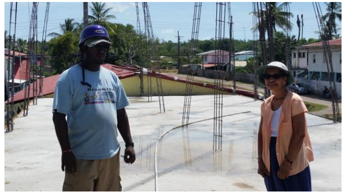
Ruth with Annoop(the contractor) on 2 nd Floor
