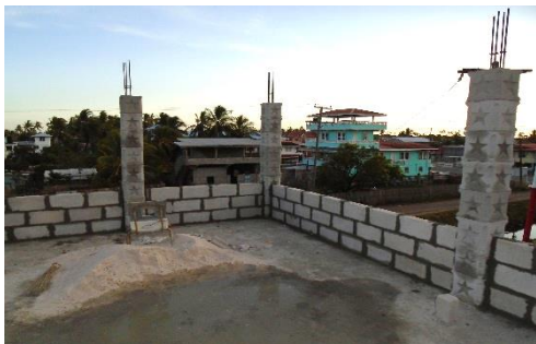
View From Veranda
