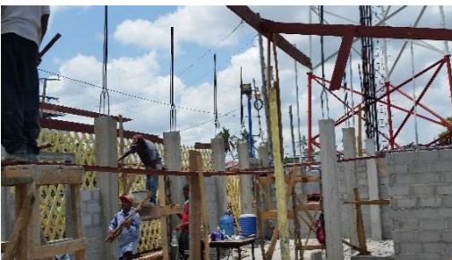
Walls Going Up
