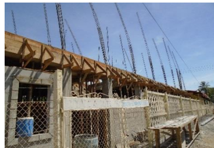
First Floor Done
