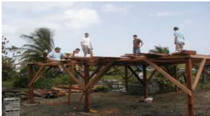
House In Progress
