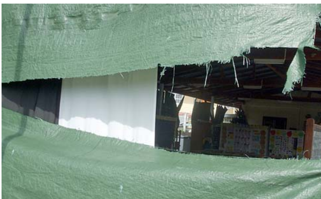
The ripped tarp under the tent.
